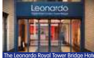
The Leonardo Royal Tower Bridge Hotel
